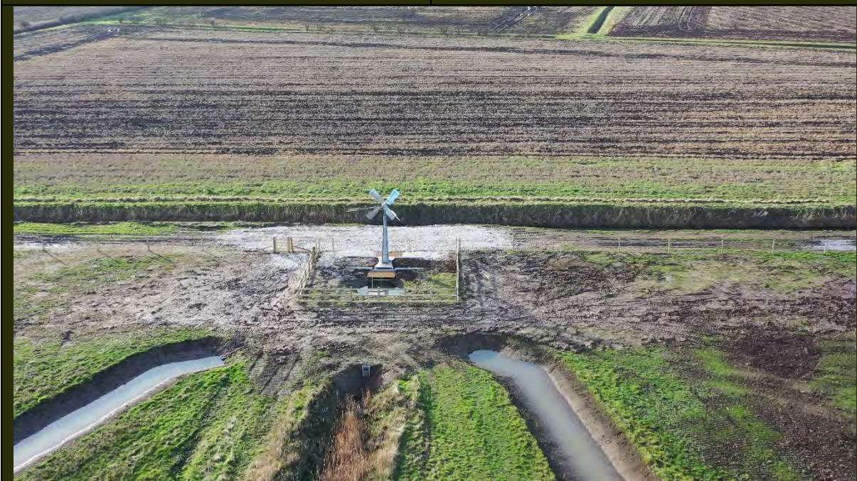
Figure 5c – Wind Pump abstracting water from Halton Drain
